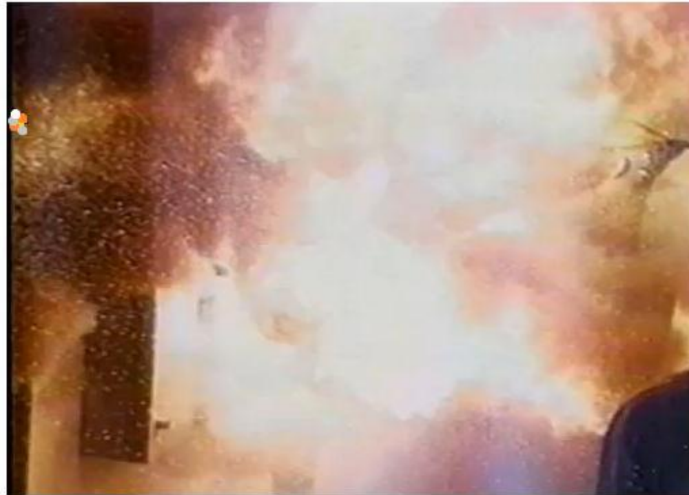
Example of an arcing fault
